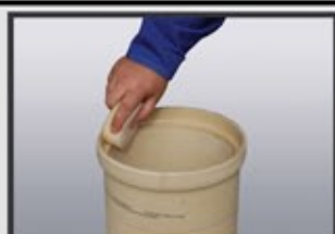
Clean the pipe edge using a moist sponge.
